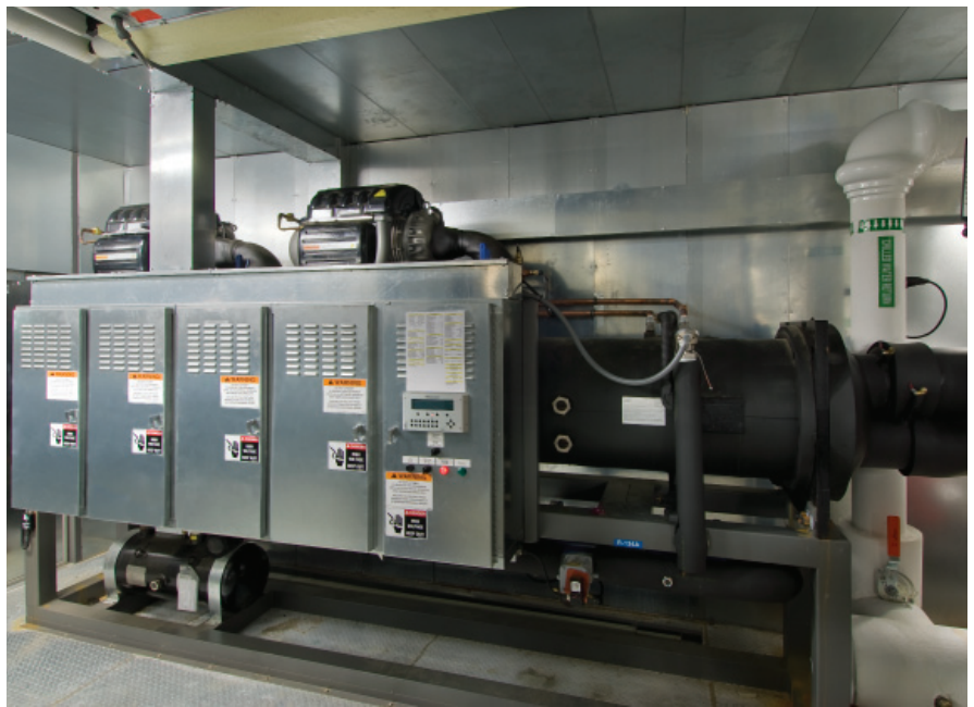
The innovative, high efficiency packaged chiller plant combines a 500-ton magnetic-bearing centrifugal chiller, evaporative condenser, waterside economizers and controls to provide the highest efficiency and low electrical demand, in addition to quiet operation and reduced maintenance and service.
