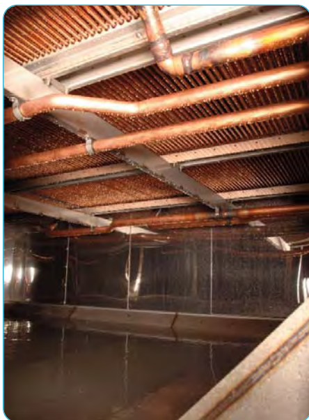
Evaporative-cooled condensers can reduce compressor energy consumption 20-40%, depending on location. Less condenser surface is required when compared to air-cooled condensers, which can reduce unit footprint as much as 50%.
