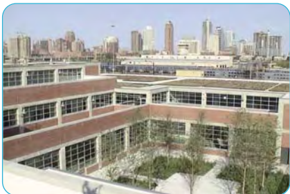
A terraced roof system aids in providing natural lighting.
