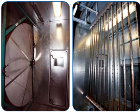
Governair air handlers encompass numerous mechanical plant functions such as energy recovery ventilation and Vapac® humidification as shown here.
