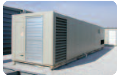
Packaged rooftop DX air-handler with integrated evaporative-cooled condenser chiller, pumps, piping, and controls
